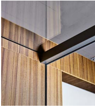
1. Junction between glass partition and wood cladding of the Bridge
