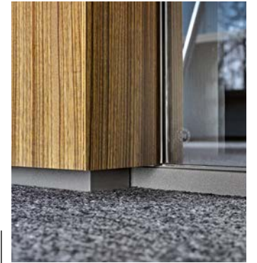
4. Junction of glass at Bridge structure showing the recessed detail
