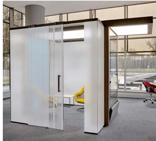
“Switchable” glass, OFF position with film on the sliding door
